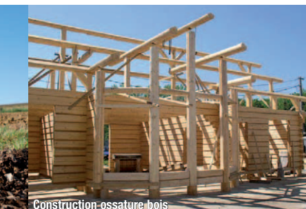
Construction ossature bois
